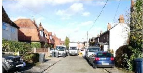
Parking on pavements in a narrow residential street
